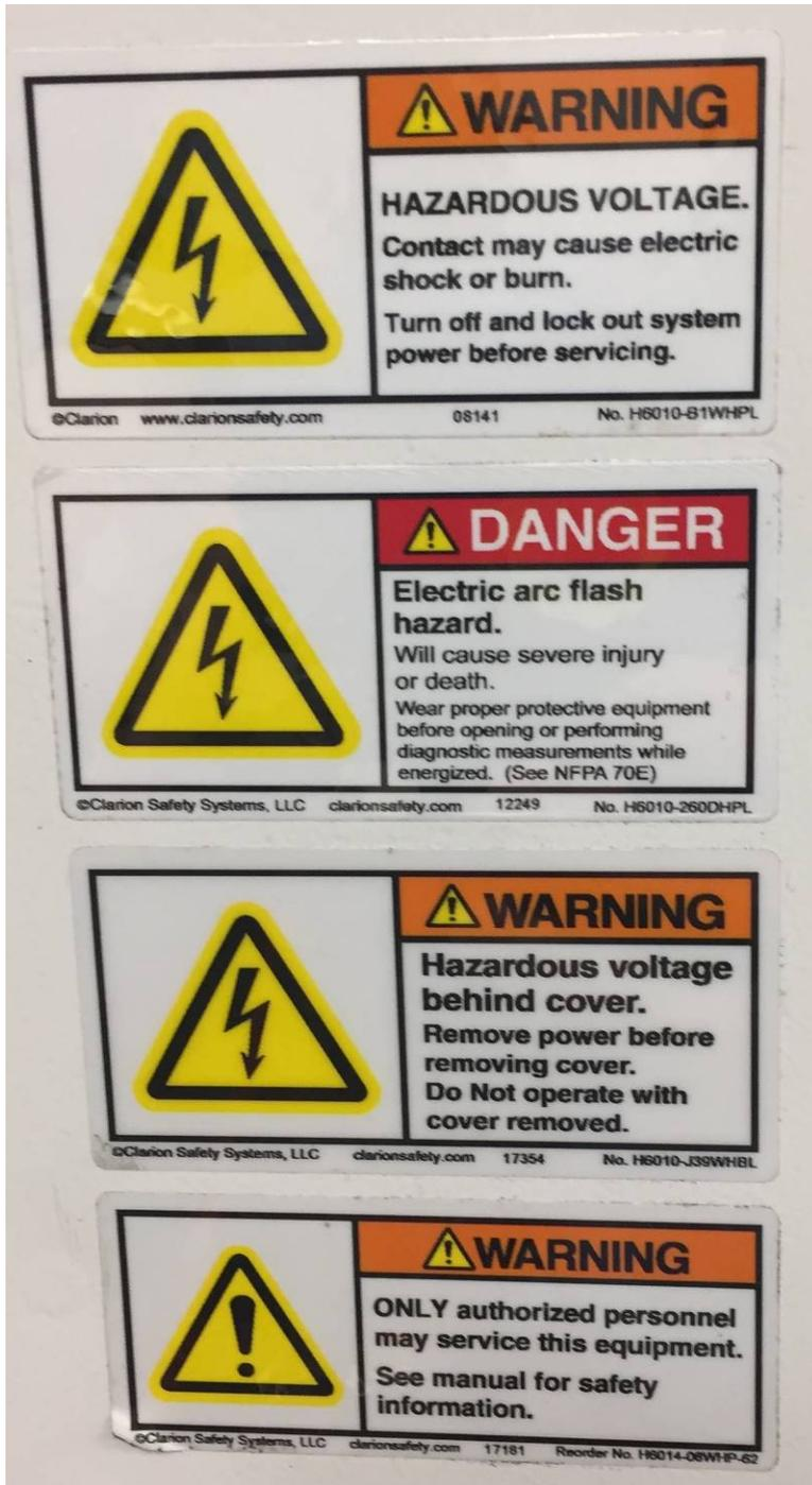
The following label located on the back of the cabinet, approximately 12” (305 mm) from the top.
