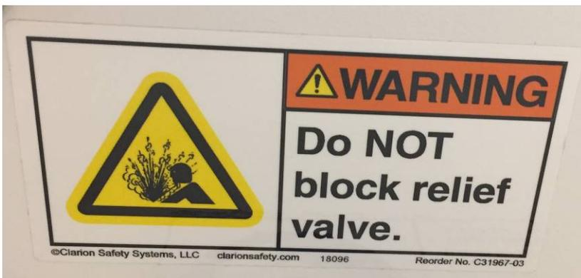
The following label is located on the GASGUARD® AP11 controller. This label is required if the GASGUARD® BSH eV System is located in a Class I, Division II rated area (United States) or in a Group 2, Category 3 ATEX rated area (Europe).
