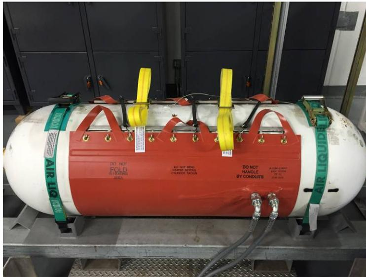
**Figure 4-10: Completed Heater Blanket Installation.**
