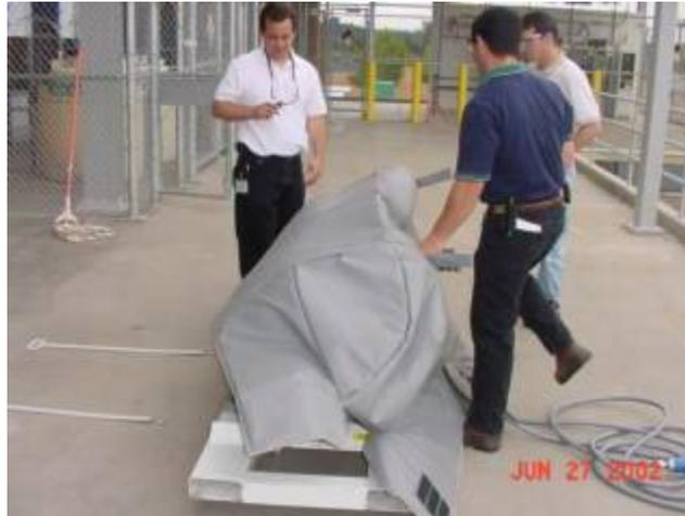
**Figure 4-12: Installation of Insulating Cover Blanket.**
