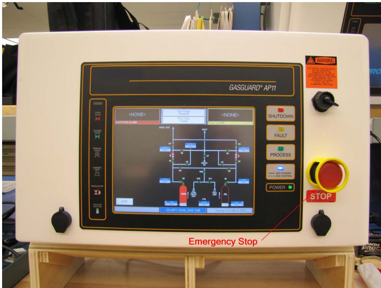
Figure 8.1: Emergency Stop Pushbutton Location
