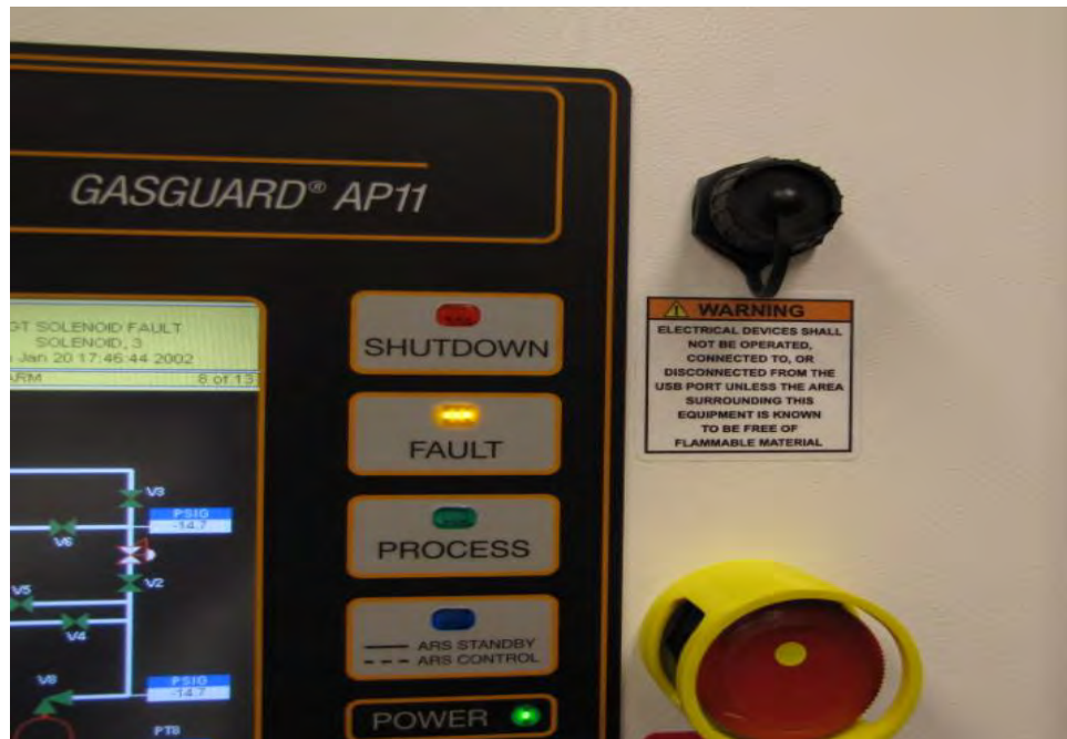
Figure 4.6b: AP11 Controller USB Port on the Face of the Controller
