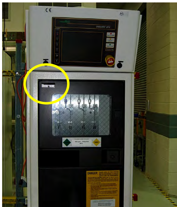
Figure 3: The AP11 Gas Cabinet equipment commodity code number (circled above) can be found on the enclosure door.
