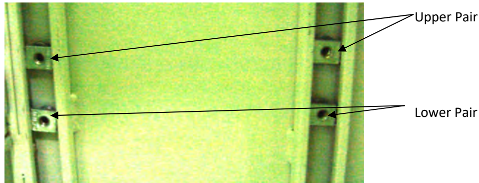
Figure 13.2.2 Unistrut nuts installed in back wall of cabinet.
