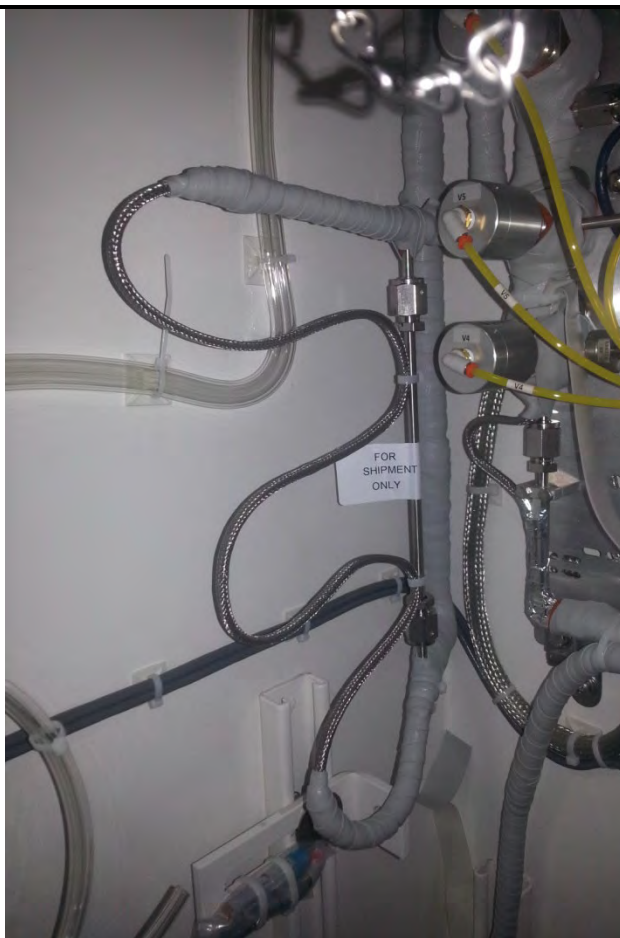
Figure 3: Service loop of heat trace cable for purifier, as shipped.
