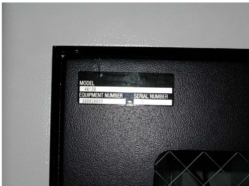
Figure 1: Equipment Commodity Code Number on a TE11 Gas Cabinet
