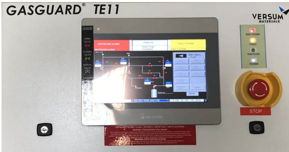
Figure 8.1: Emergency Stop Pushbutton Location
